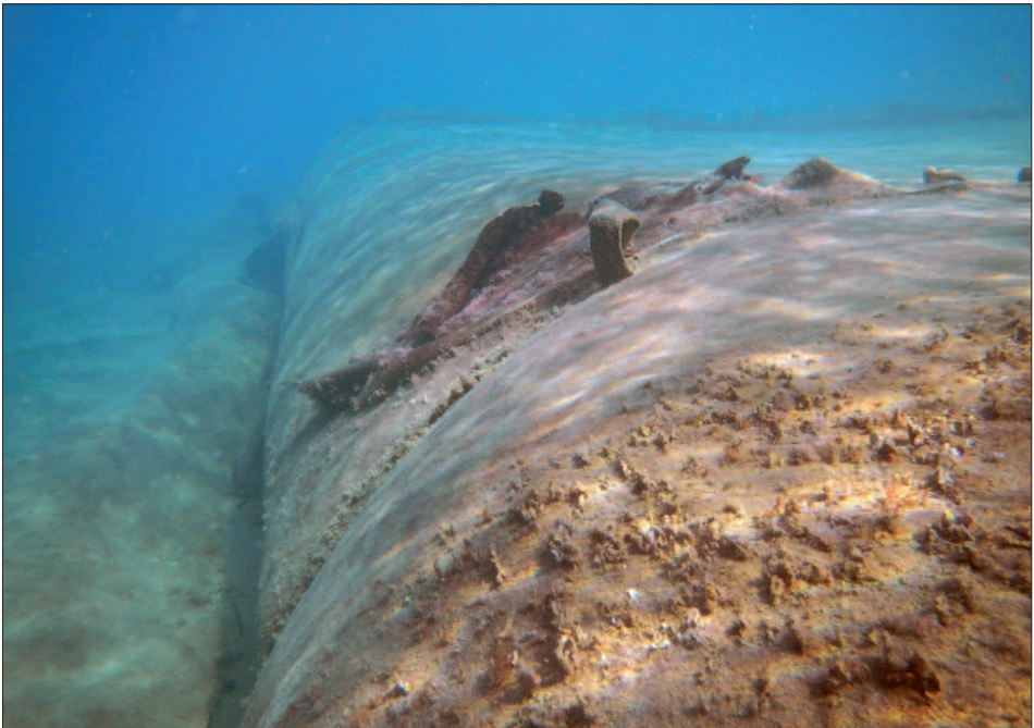
Figure 3 - Submerged artificial breakwater made of geotextile at San Vincenzo (Livorno).
