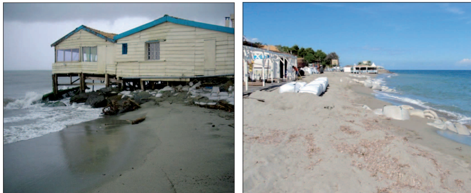
Figure 16 – Coastal erosion trends at Tavignano. a) Beach restaurants endangered by shoreline retreat (October 2007); b) Engineering solutions executed to protect a camping site and economic activities on the backshore (September 2010).
