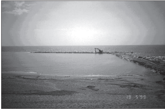
Figure 15 - Above: works executed on 19 05 1999 (Photo: DST-UNIFI archives); Right: structure status on 13 03 2000 (Photo: Corpo delle Capitanerie di Porto, Luni - Sarzana). Although the structure was designed with a submerged crest, it induced changes on beach morphology that had not been predicted by the project.
